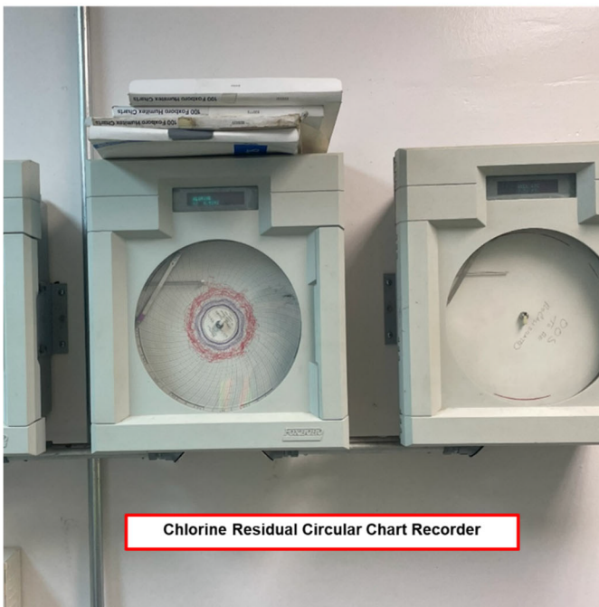
Figure 2-4 Sample Chlorine Monitoring Equipment
